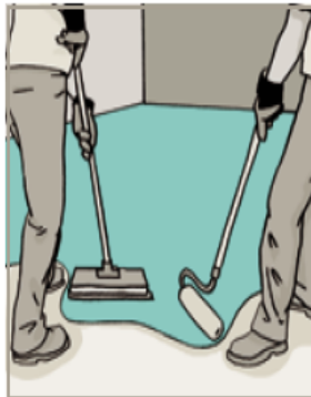
Apply the coating in the required layer thickness.
