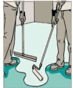
Apply the seal coat using a squeegee and roller.
